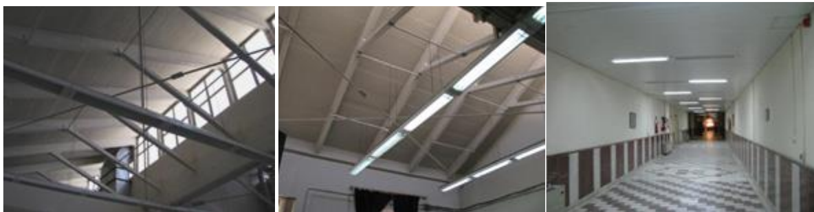
Fig. 7. A view of the Pashmina building after its renovation; its unique structural system has remained out of sight as its aesthetic and identity characteristics.
