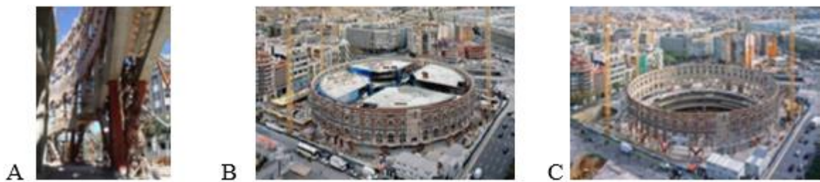
Fig. 4. a. Reconstruction of the historic shell with new sections, b. Attachment and repair of the façade, c. Reinforcement of the facade and foundations, separation of additions.
