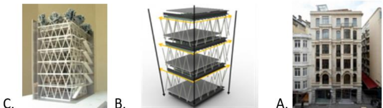
Fig. 8. A. Historical shell of the Bursan Music and Art House (2010 As), b. Project structural model C. Project structural component model.
