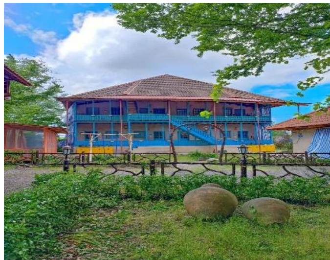
Fig. 2. The Gholam-Gardesh pattern and open circulation system in vernacular architecture.
